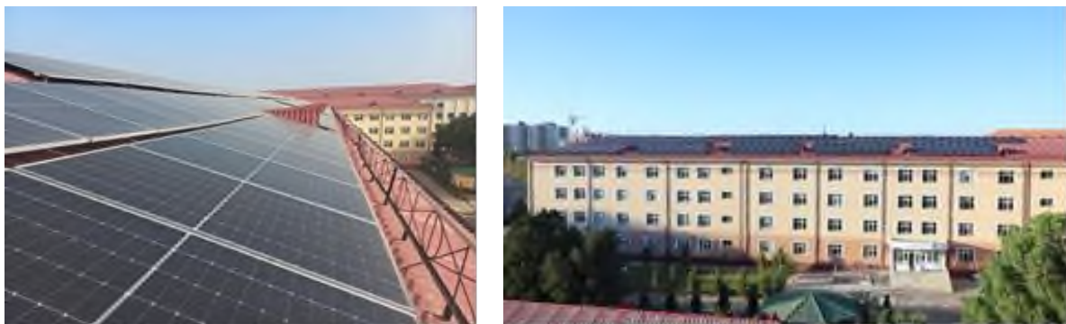
Figure 1. Overview of on-grid solar system.
